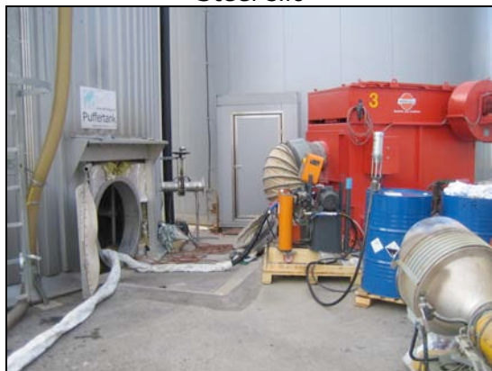
Placement of spray-machine
